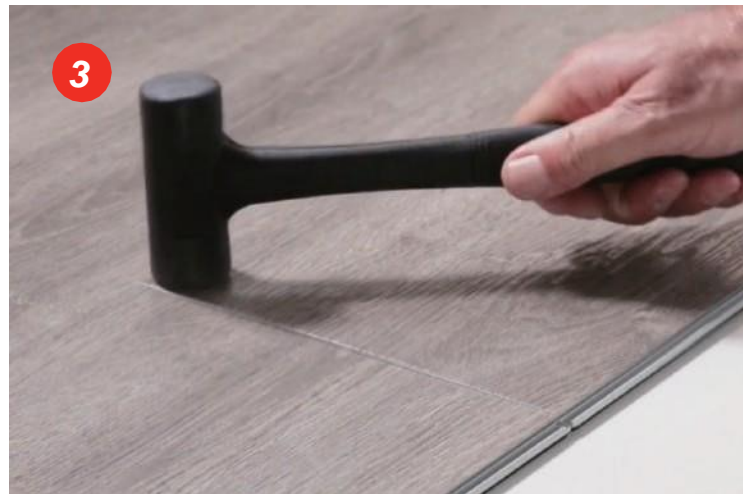
Use a soft-faced hammer to lock the planks on the short side
