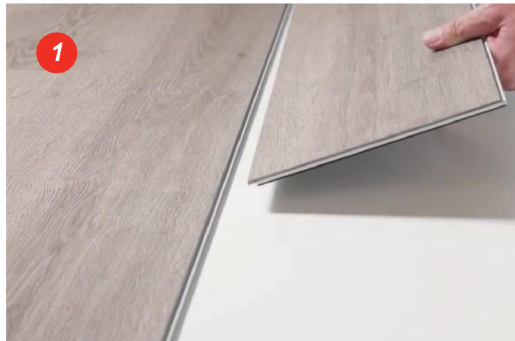
Connect the long side at an angle
