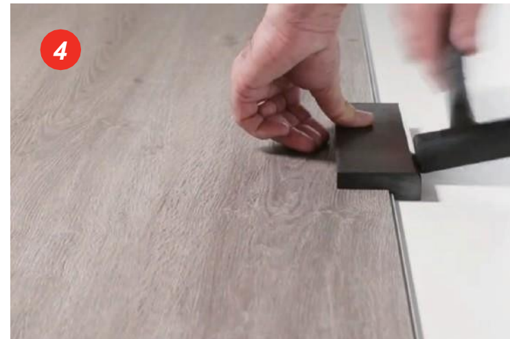
Use a soft-faced hammer to properly lock the planks
